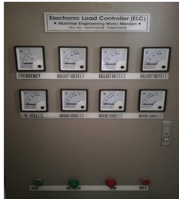
Figure 3-13: Electronic Load Controller Assembly (Mukhtiar Engineering)
