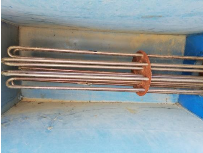
Figure 3-15: Dummy Load: Water Heater
