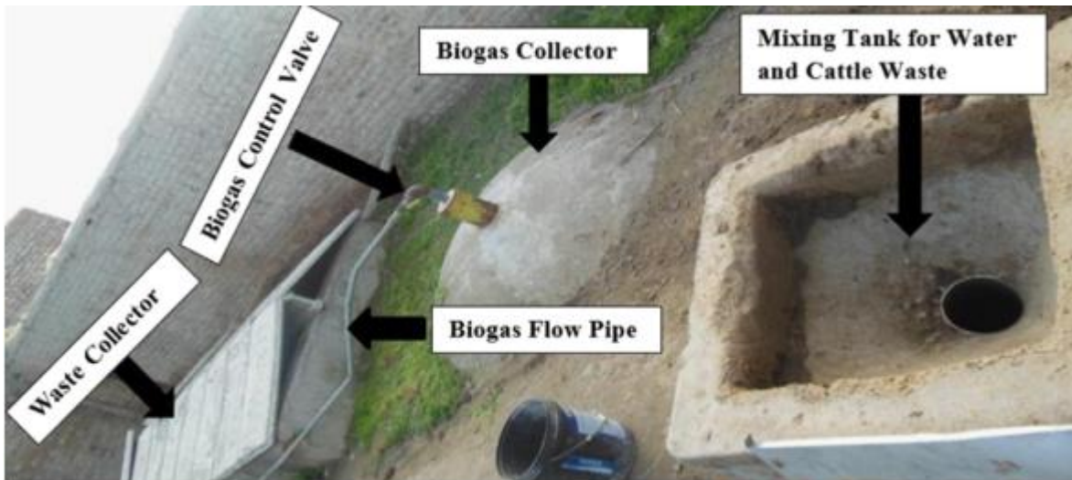
Figure 4-13 Fixed Dome Biogas Digester [12]
